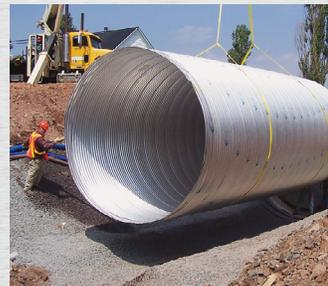
For more corrosive environments, Aluminized Type 2 coating offers the superior corrosion resistance and surface characteristics of aluminum with the strength and economy of steel. In this
