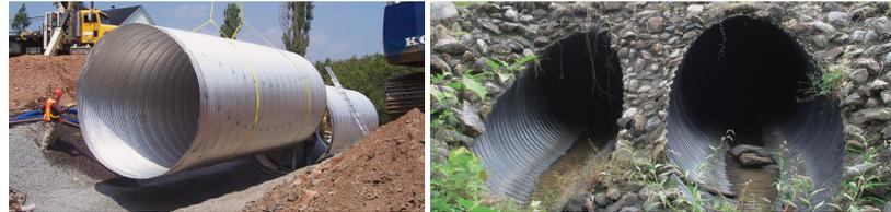
It will not crack under impact loads or vibrations due to the inherent strength of steel and the flexibility of the corrugated pipe section. The high ring compression of the pipe absorbs and transfers the load to the surrounding soil around the entire circumference. The beam strength maintains the grade and line of the structure by bridging inequalities of the trench bottom and side fill.
