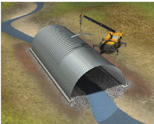
If specified, reinforcement ribs are then added.
