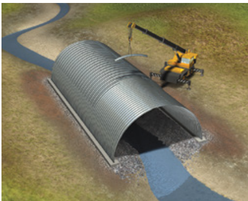
If specified, reinforcement ribs are then added.
