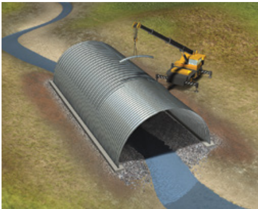
If specified, reinforcement ribs are then added.
