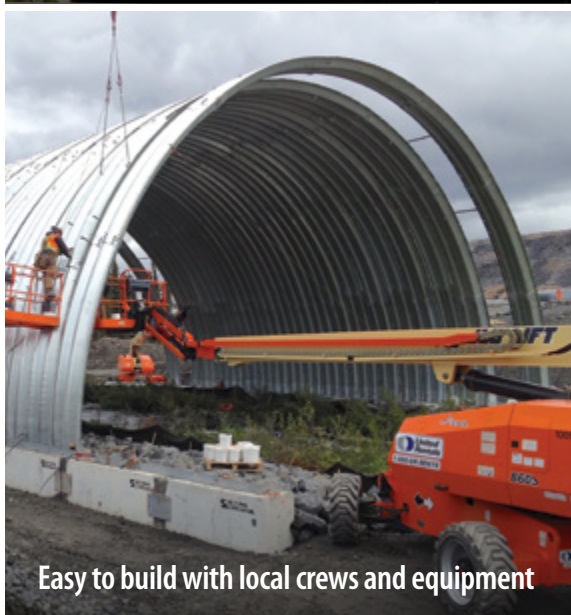
Stream crossing for military base designed to support heavy-duty tanks and equipment
