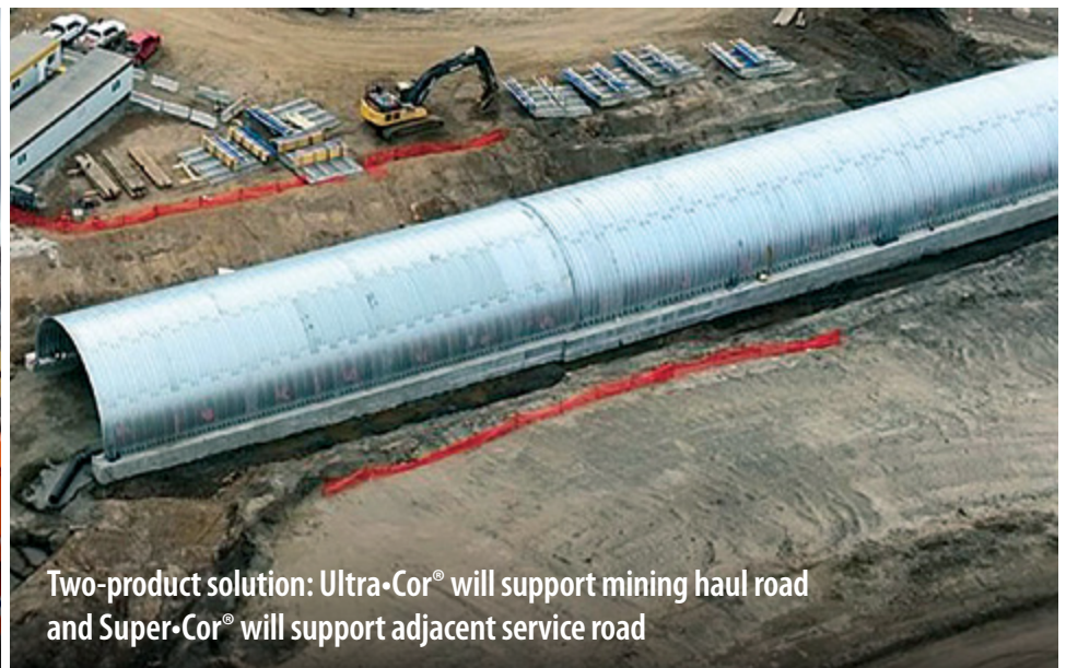
Mining haul road crossing under construction
