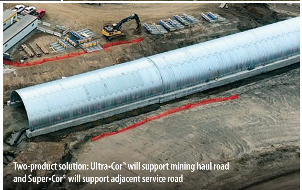
Mining haul road crossing under construction
